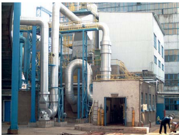
FIG. 1. Pilot plant for electron beam flue gas treatment at the Maritsa East 2 thermal power plant in Bulgaria.
